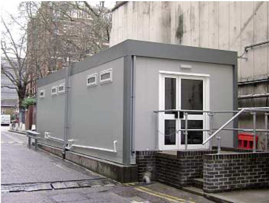
The CompPod's compact dimensions enable it to occupy only a small footprint. Over 1 tonne of food waste from multiple producers on site is composted here every week.
